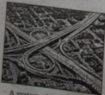
A system of expressways with overpasses
